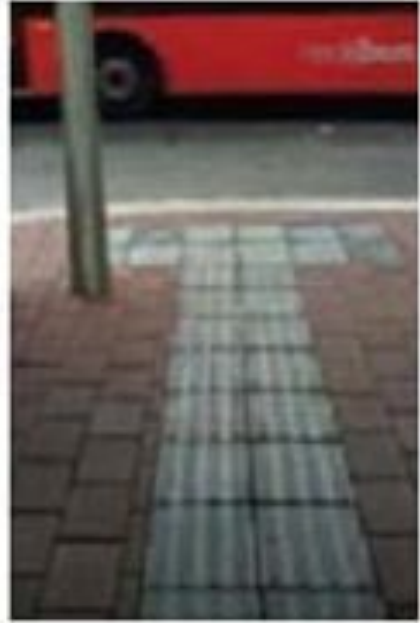
Example of TGS installation
