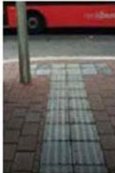
Example of TGS installation
