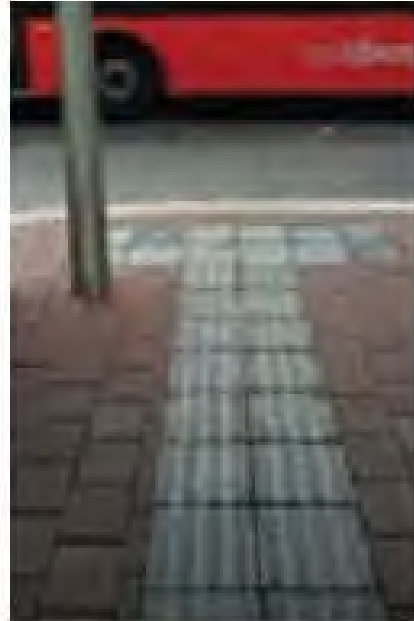
Example of TGS installation
