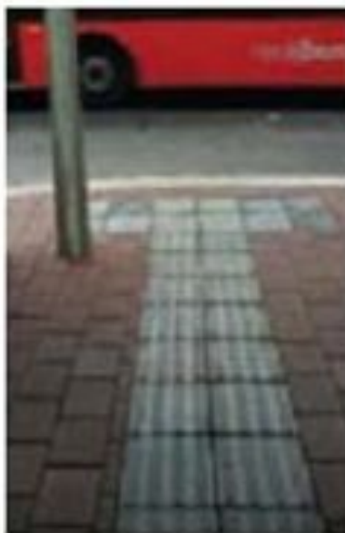
Example of TGS installation
